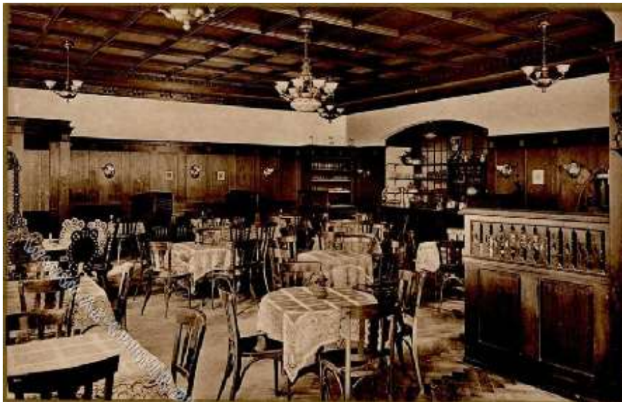
City (Excelsior) Hotel, Sihlstr. 7/9, 8001 Zürich
